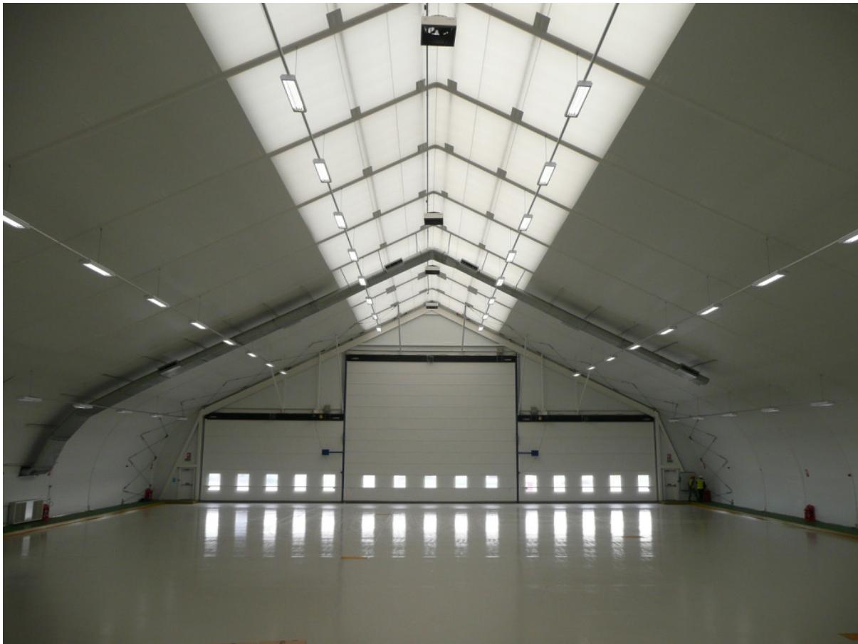
Viewing window into Hangar from office structure
