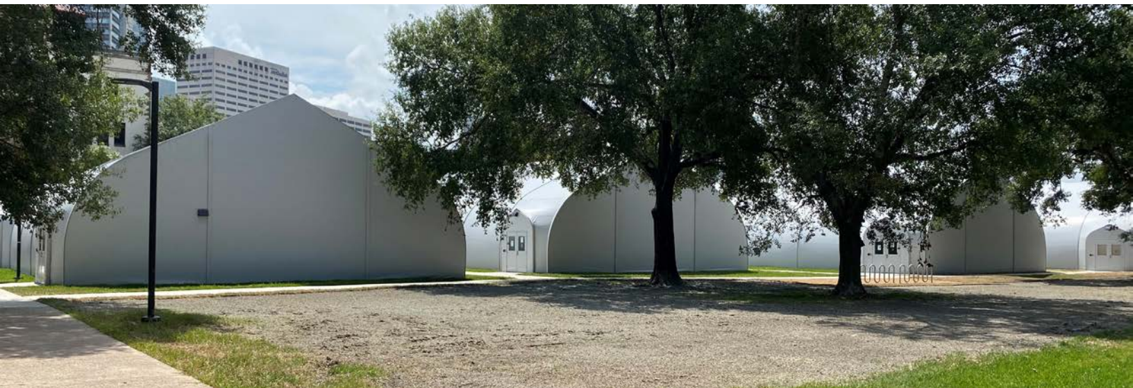
Four insulated structures feature audio-visual technologies and HVAC for comfortable and functional learning.
