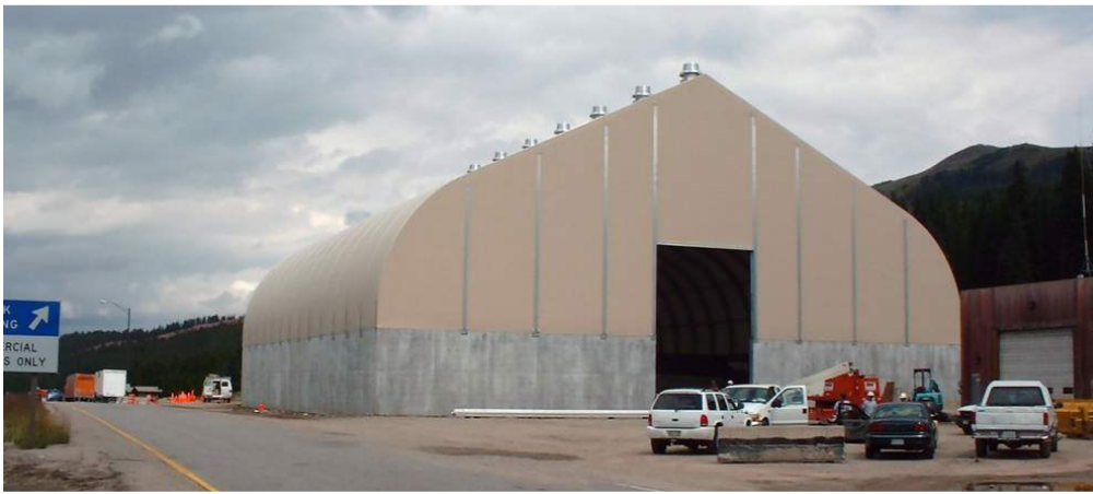
Salt/Sand Storage Facility Vail Pass, Colorado Rockies
