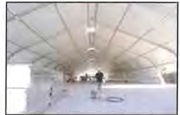
Gov. Linda Lingle's plan to ease the housing shortage on the Leeward Coast includes a temporary transitional shelter under construction near Wai'anae Intermediate School.
